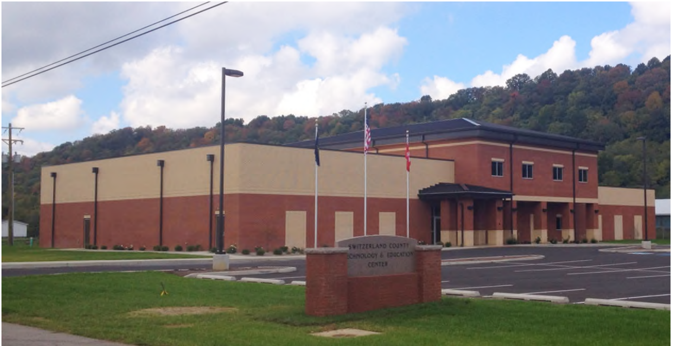
Switzerland County Technology and Education Center
